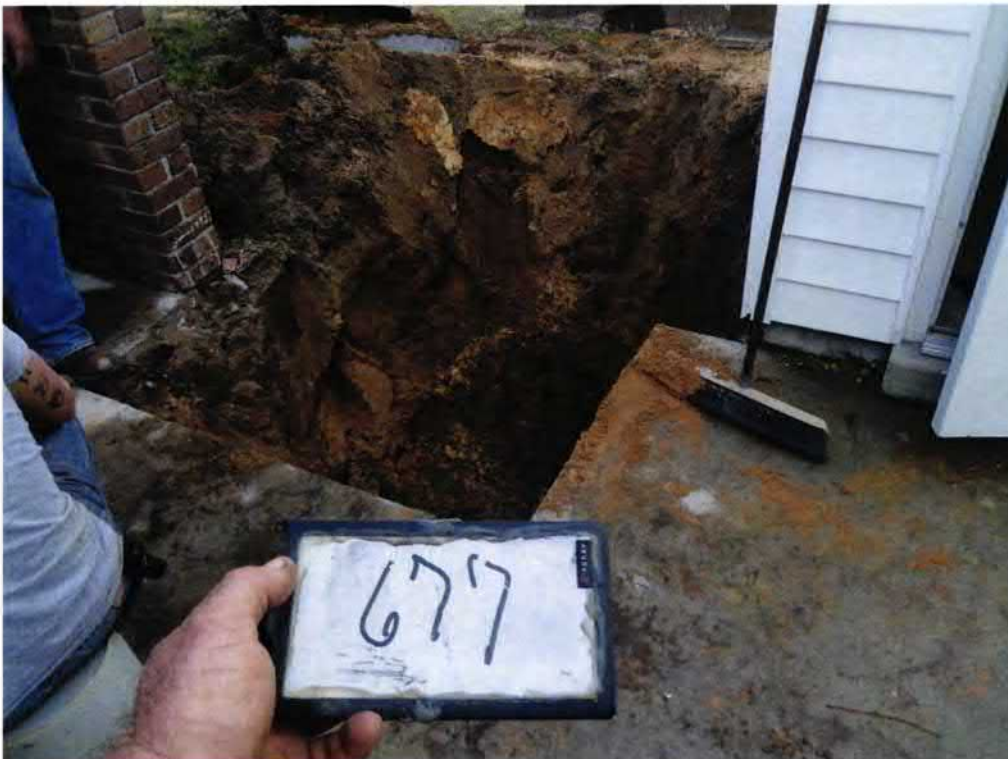
Picture 2: UST 677Camellia excavation.
